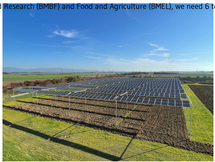
In elevated solar panels, the photovoltaics (PV) modules are located at least 2.1 metres above ground level. This allows the area below the solar modules to be used for agricultural purposes. For ground-mounted solar panels, the areas between the modules are typically used for farming. © Krinner-Carport GmbH
