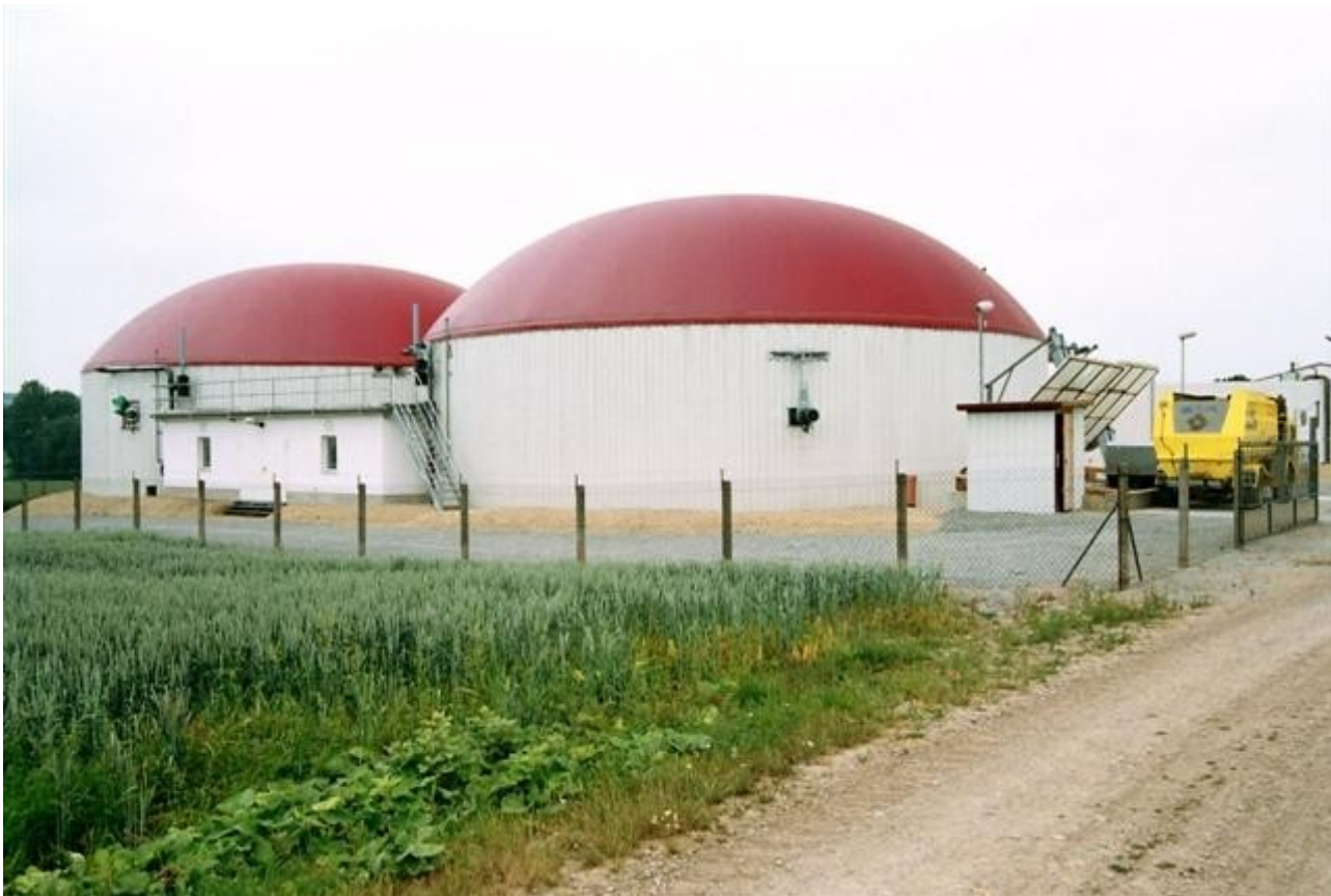
Biogas plant. © BMU
