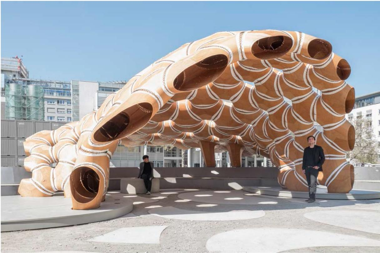
The research pavilion at the University of Stuttgart campus is based on a lightweight scaffolding structure made of thin veneer panels that are sewn together by robots<sup>9</sup>.
