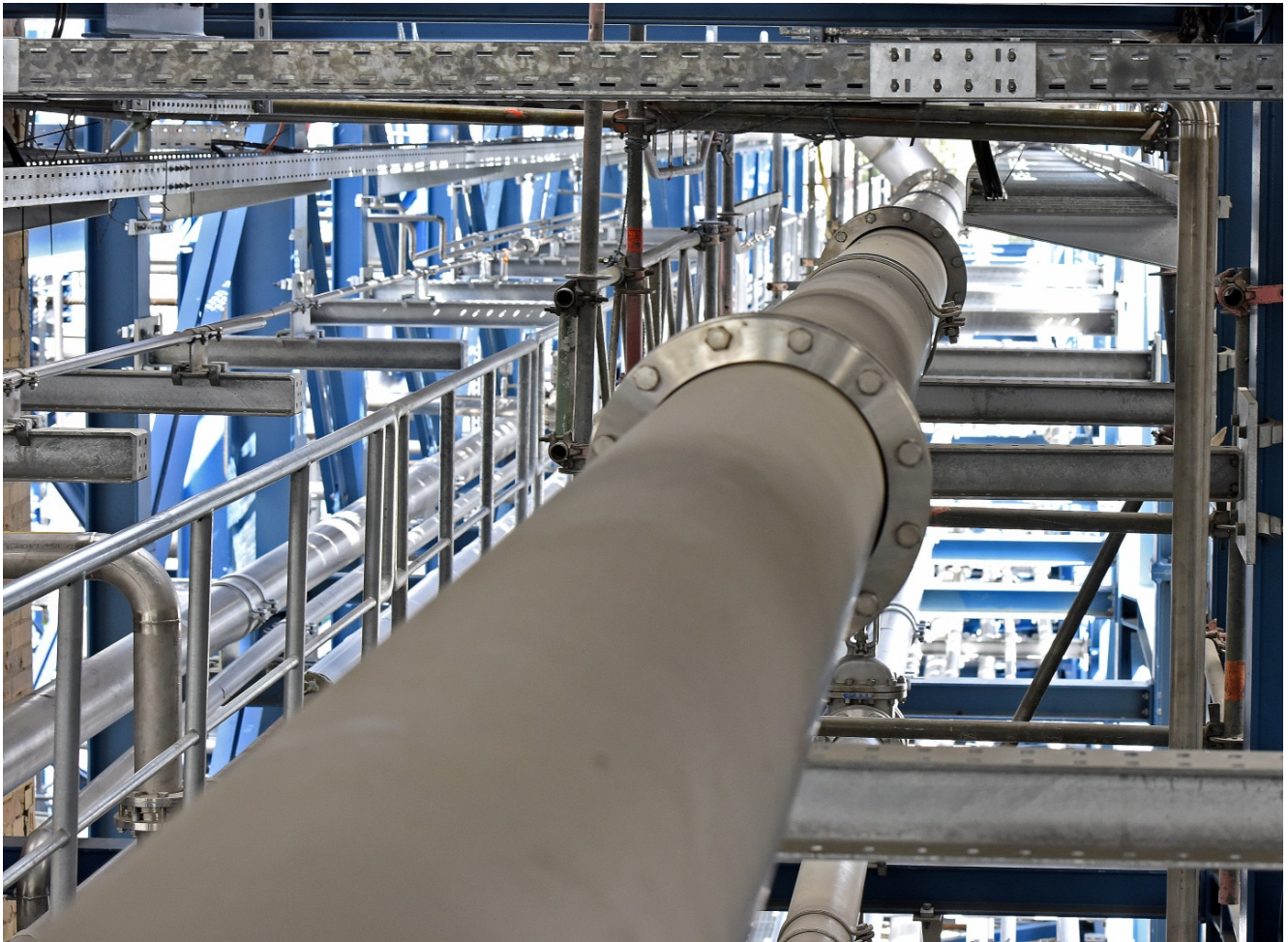
The liquid pulp is transported to the paper machines via a pipeline more than 1 km long. © Essity/Tröster
