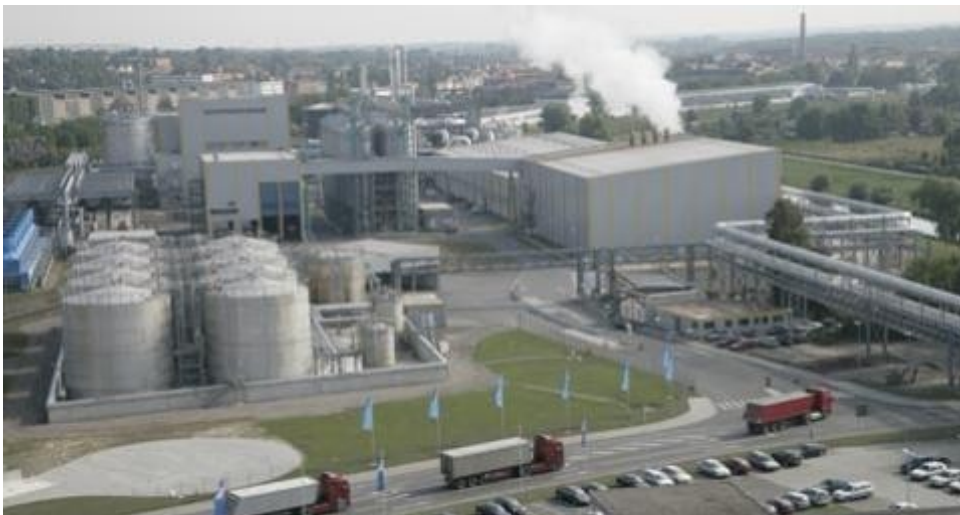
Bioethanol-Anlage Zeitz © CropEnergies AG
